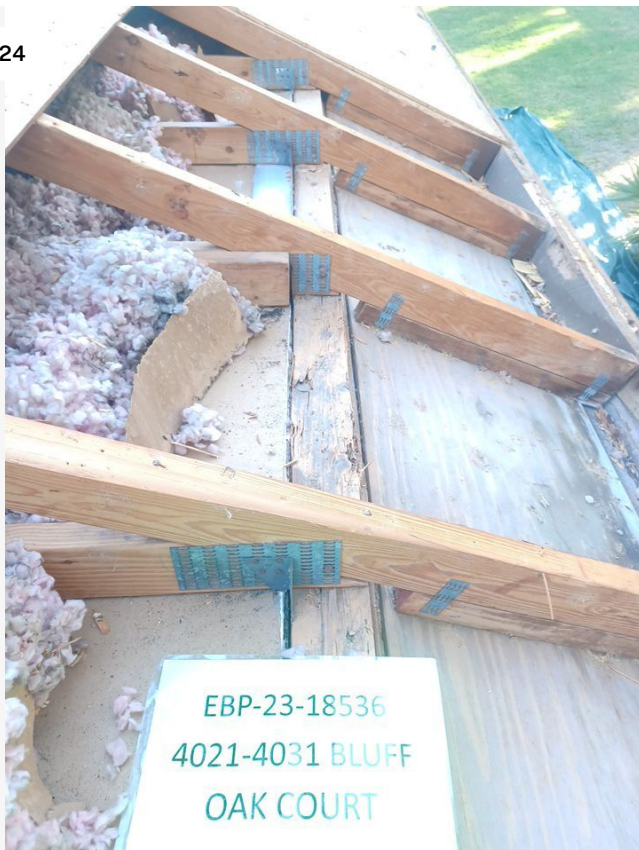
Project: STRATHMORE GATE - 4021-4031 BLUFF OAK CT / 2310-5005438-01 Date: 11/27/2023, 3:53pm Creator: Lucio Roofer
