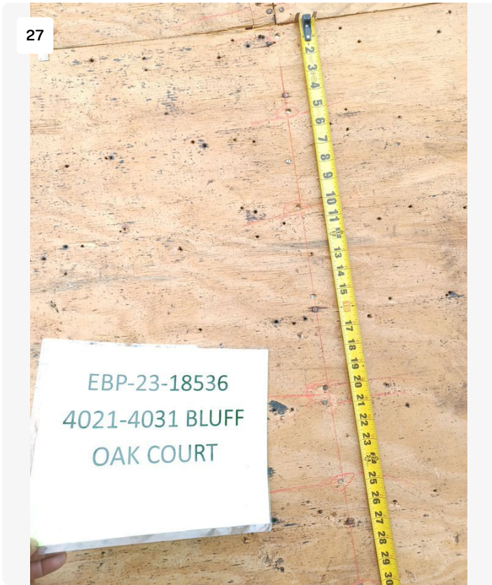
Project: STRATHMORE GATE - 4021-4031 BLUFF OAK CT / 2310-5005438-01 Date: 11/28/2023, 1:53pm Creator: Lucio Roofer
