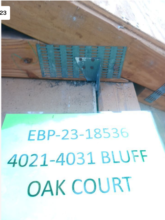
Project: STRATHMORE GATE - 4021-4031 BLUFF OAK CT / 2310-5005438-01 Date: 11/27/2023, 3:51pm Creator: Lucio Roofer
